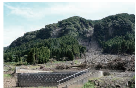
Damage from torrential rains in Kyushu (Aso, Kumamoto)
